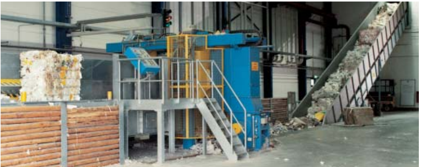
Fig. 2: Waste paper charging system with automated bale dewiring, designed and built by B+G Fördertechnik GmbH, Euskirchen, an associated company of Voith Sulzer Paper Technology Group.
