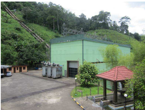
The Polpitiya power house (source: Voith Hydro GmbH & Co KG)
