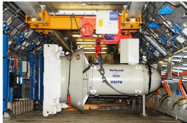
Figure 3 StreamDiver® on crane hook before installation
