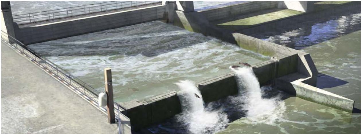
Fig. 5: Overflowed plant with fish migrating downstream over gate
