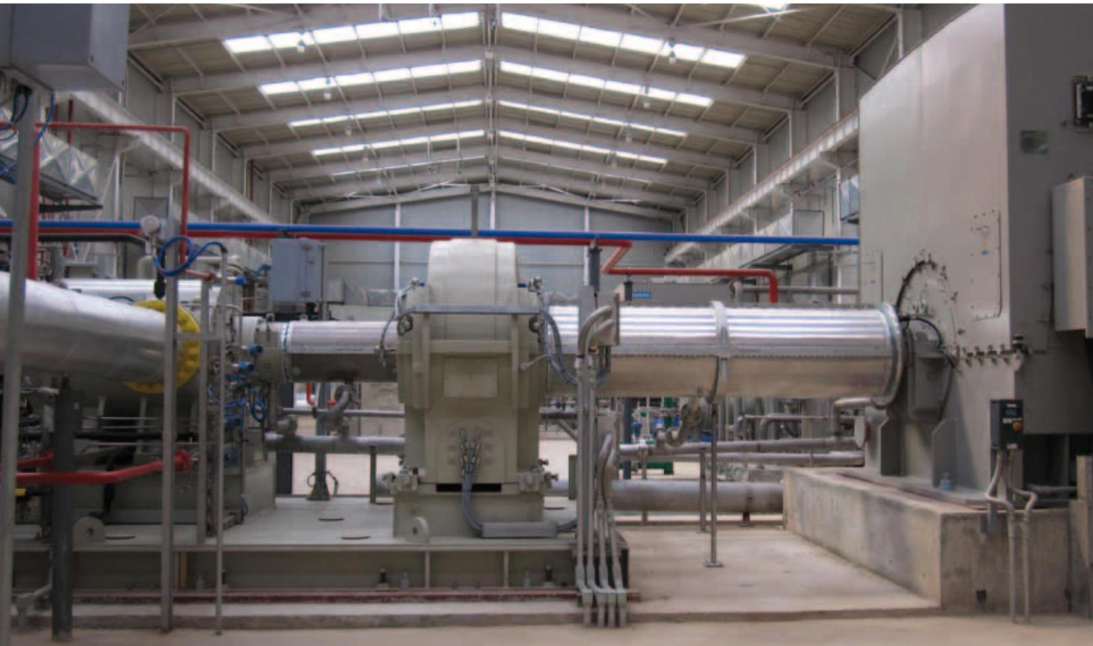
Figure 5: Voith Turbo BHS parallel-shaft gear unit in compressor station at YangQu for the Shaanxi to Beijing pipeline of PetroChina with 20,000 kW power, input speed 1,800 rpm, output speed 8,594 rpm.
