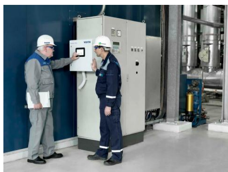
Figure 1: Bilfinger Maintenance Nord has chosen the new TurCon DTm turbine controller from Voith as part of a tandem turbine upgrade at the UPM paper factory in Ettringen. The high degree of flexibility, simple parameterization and easy to use operating concept make the digital controller a compelling choice.
