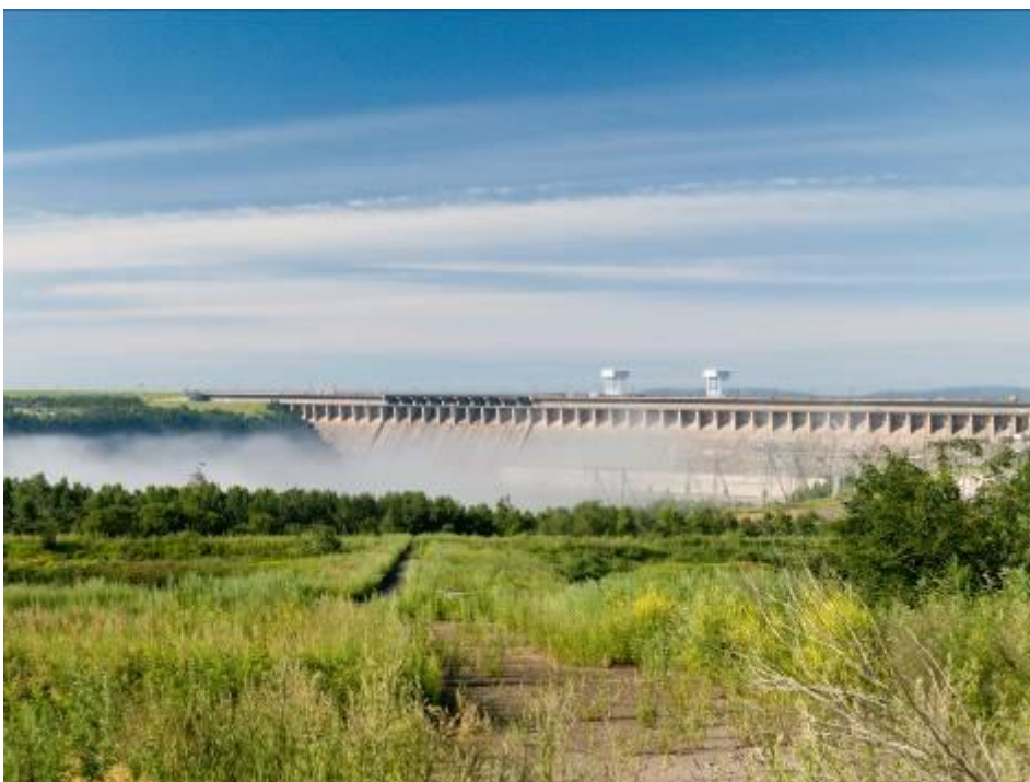
Bratsk hydro power station (Source: Irkutskenergo)
