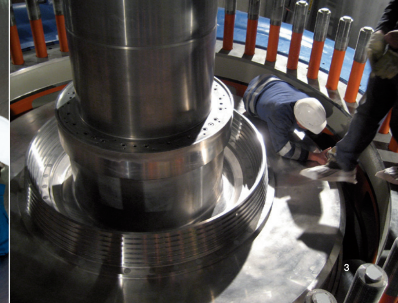
3 Assembly of the runner, final stage, Kops II, Austria
