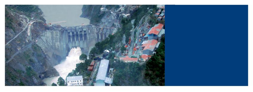
Baglihar stage-I & Stage-II (each of 3x150 MW) Hydro Electric Projects owned by Jammu & Kashmir State Power Development Corporation is run of the river project on Chenab River in State of Jammu & Kashmir, India. The water for both the stages shall be fed from common barrage.
