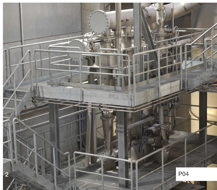
2 HiPRO Protector System installation
