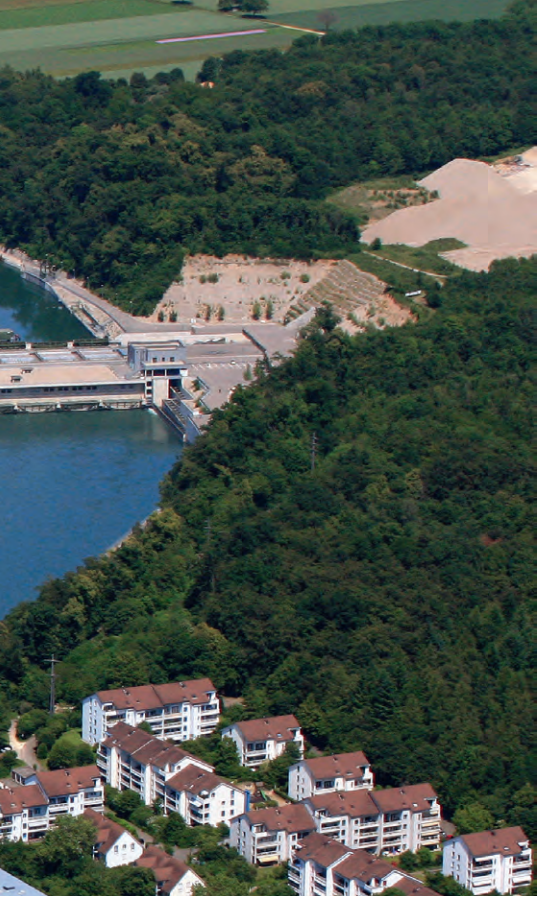
The Rheinfelden run-of-river power station. The new power plant was built from 2003 to 2010
