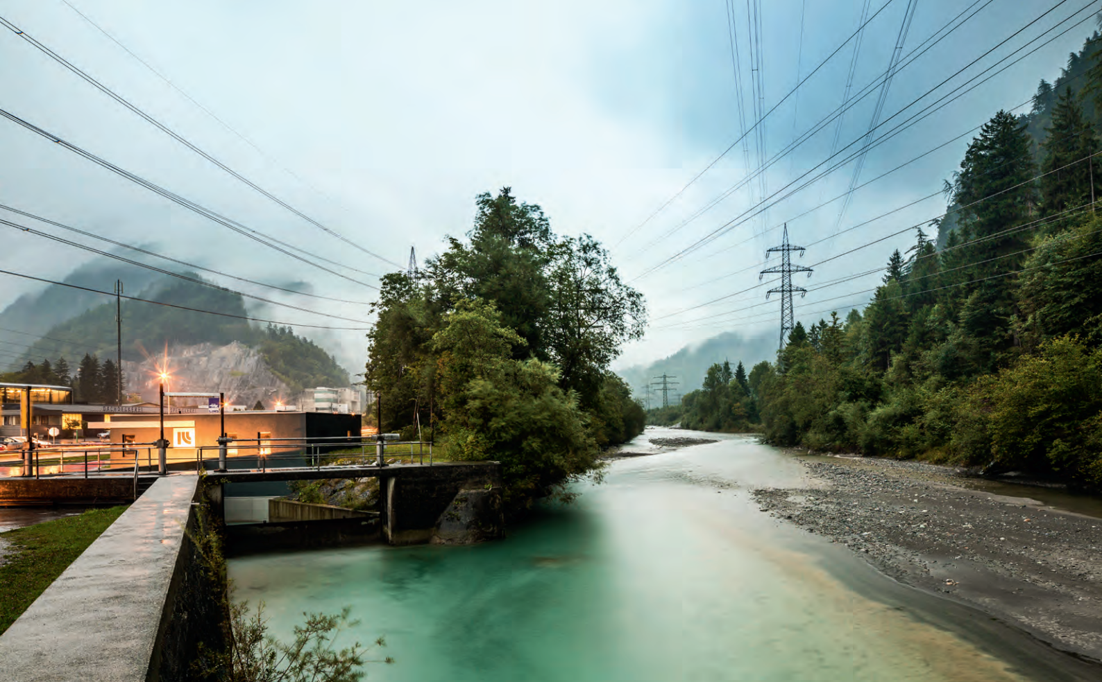
The small power station at Brunnenfeld supplies energy to 360 homes
