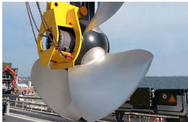
Fitting of a turbine for the run-of-river power station, Rheinfelden
