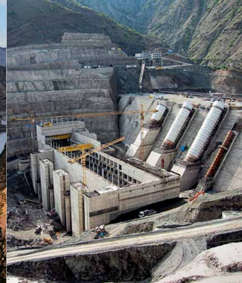
Beyhan I is the first of four hydropower plants in this area of the Murat river. Voith Hydro is fitting the plant with three generators.
