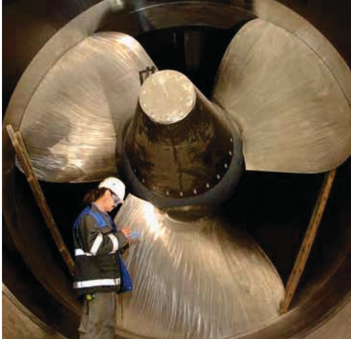
The largest of their kind in Europe: the Kaplan pit turbines at Litoměřice
