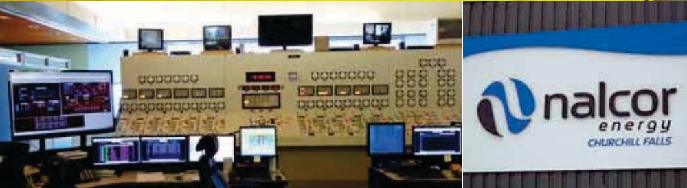
After about 40 years of service, CF(L)Co decided to replace control systems at Churchill Falls. Electronic automation will enable optimized operation thanks to more available information.
