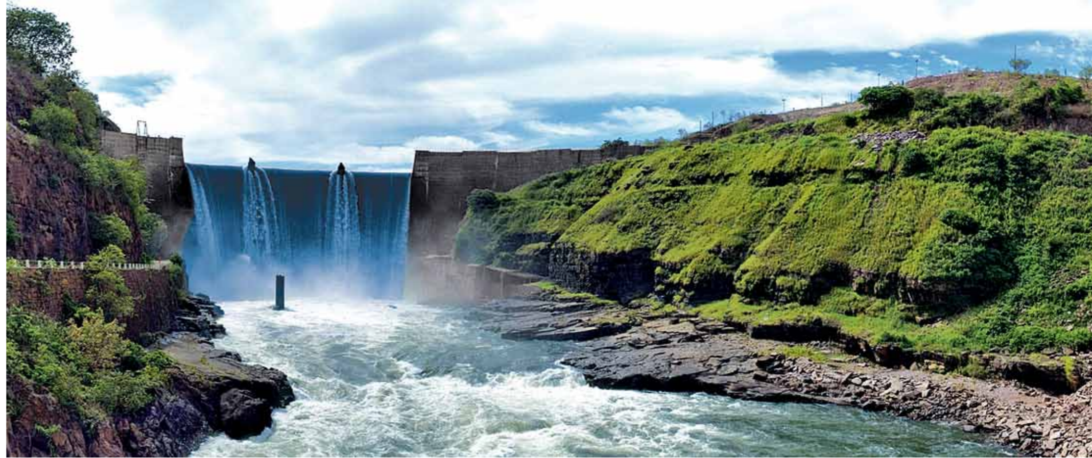
Voith has completed a major upgrade of the Cambambe plant on the Kwanza River. Now, a second plant is planned for the region.
