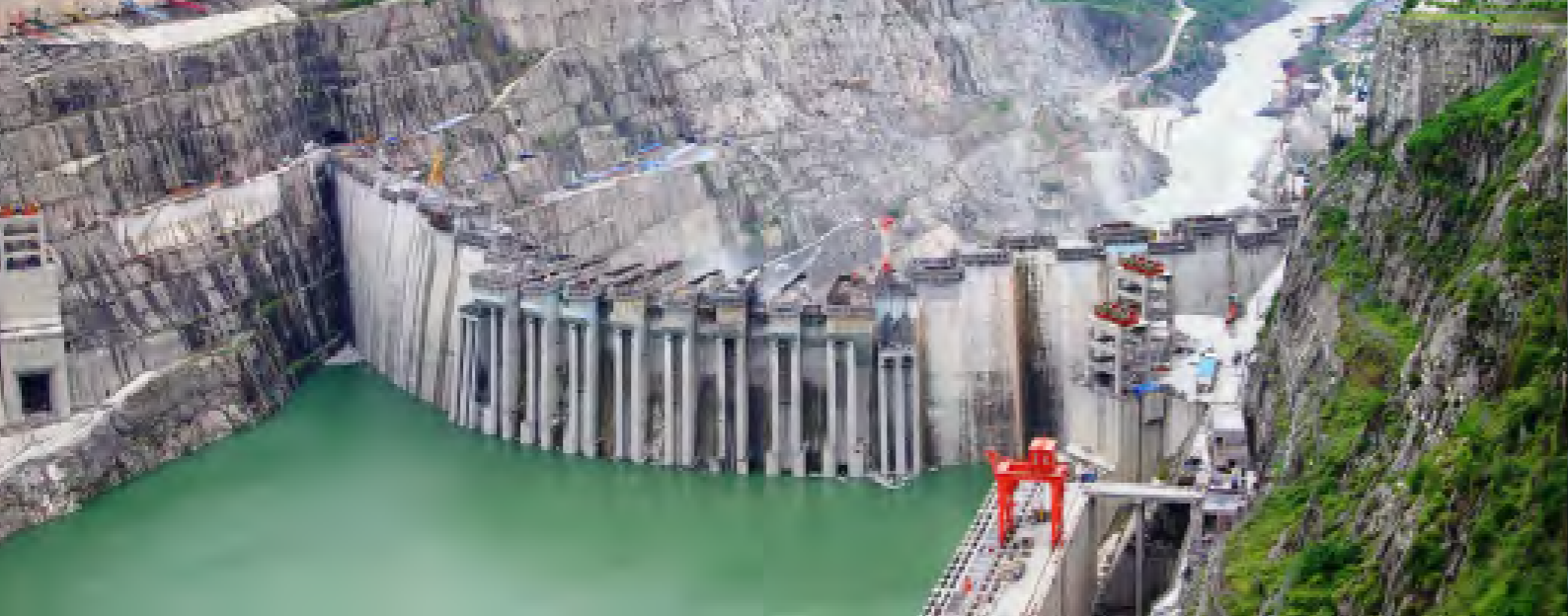
Plant under construction, Xi Luo Du, China
