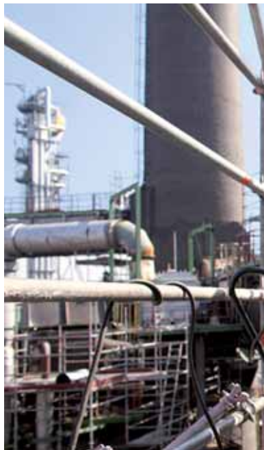
Mechanics from Voith Industrial Services carrying out maintenance work at a refinery.
