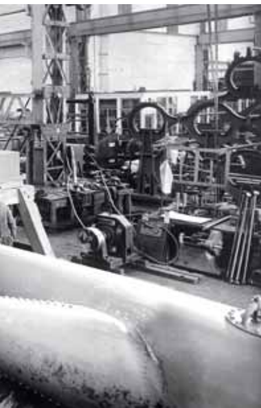
Between 1903 and 1912, Voith delivers 12 Francis twin turbines for the Ontario Power Company power station at Niagara Falls.
