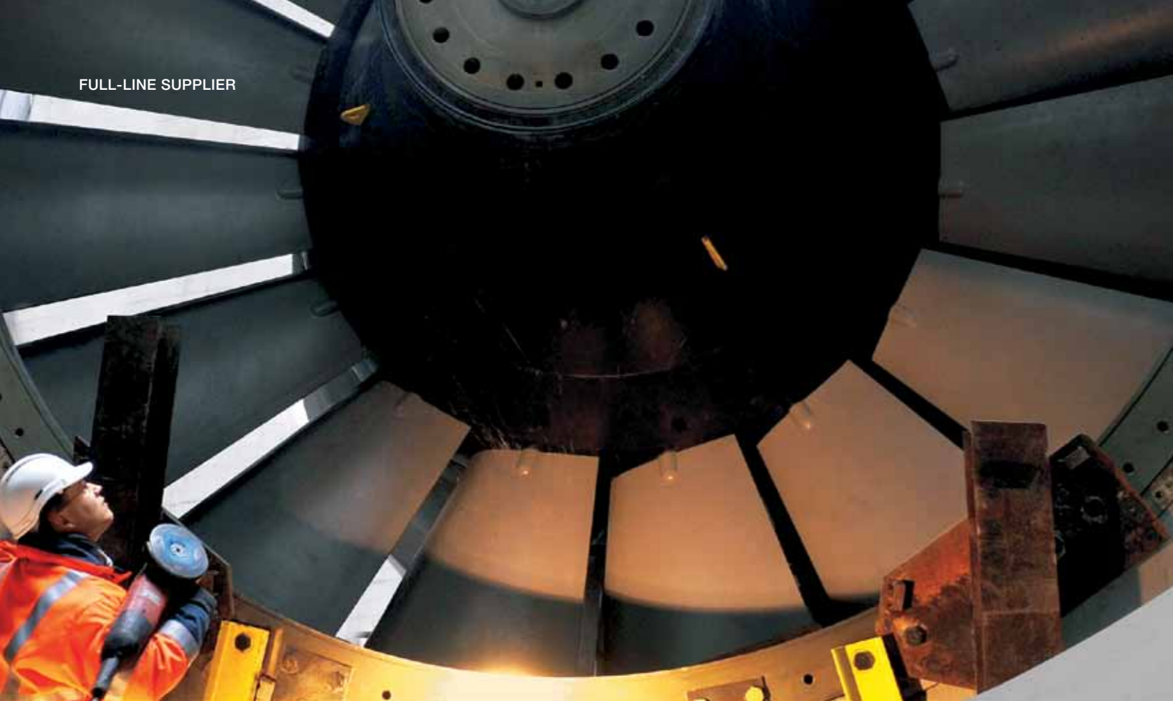
Guide vane for the equipment of the completely rebuilt Rheinfelden plant at the Swiss-German border.
