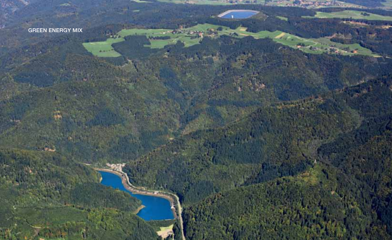
Aerial view of the lower and upper reservoirs at Wehr, southern Germany.
