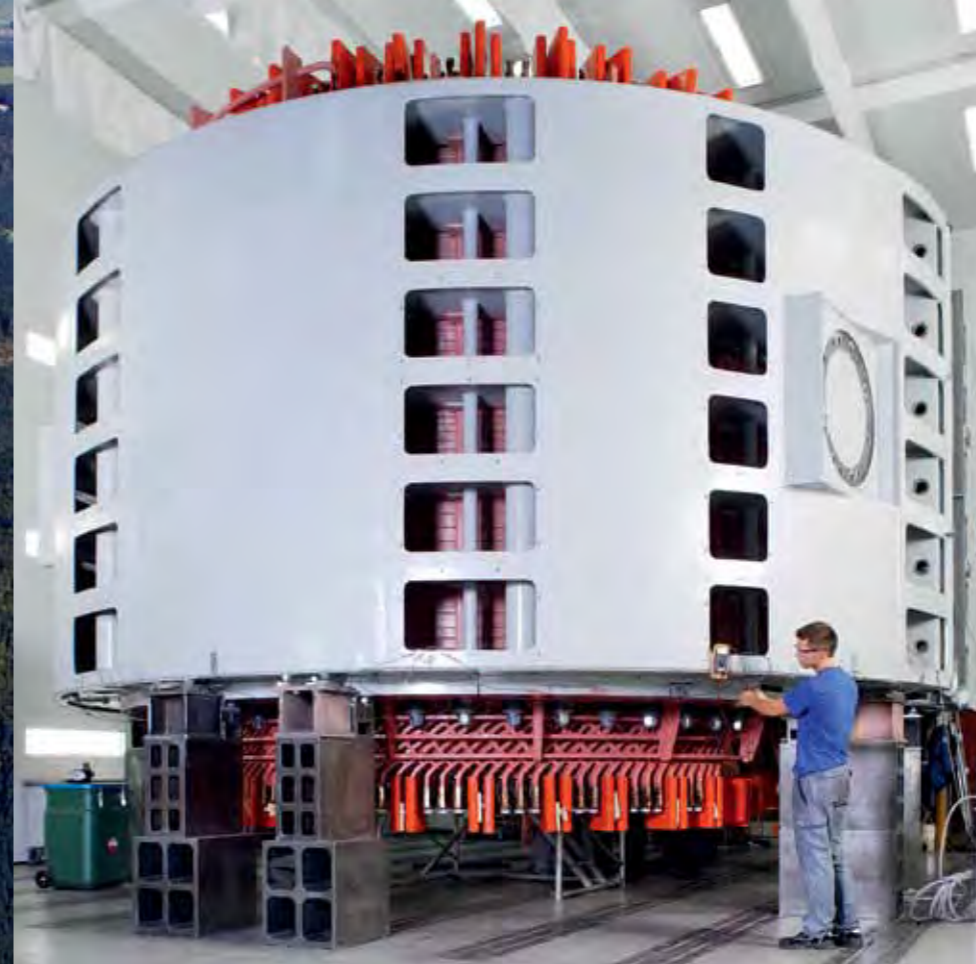
Modernization work carried out on one of Wehr's generators.
