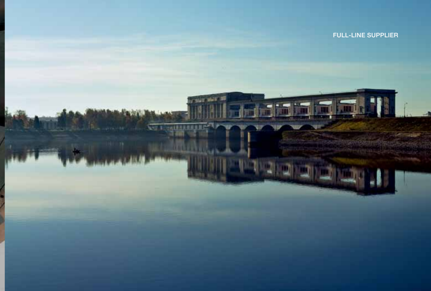
In Uglich, Russia, Voith Hydro carried out extensive modernization work, boosting the unit's capacity by almost 20 percent.
