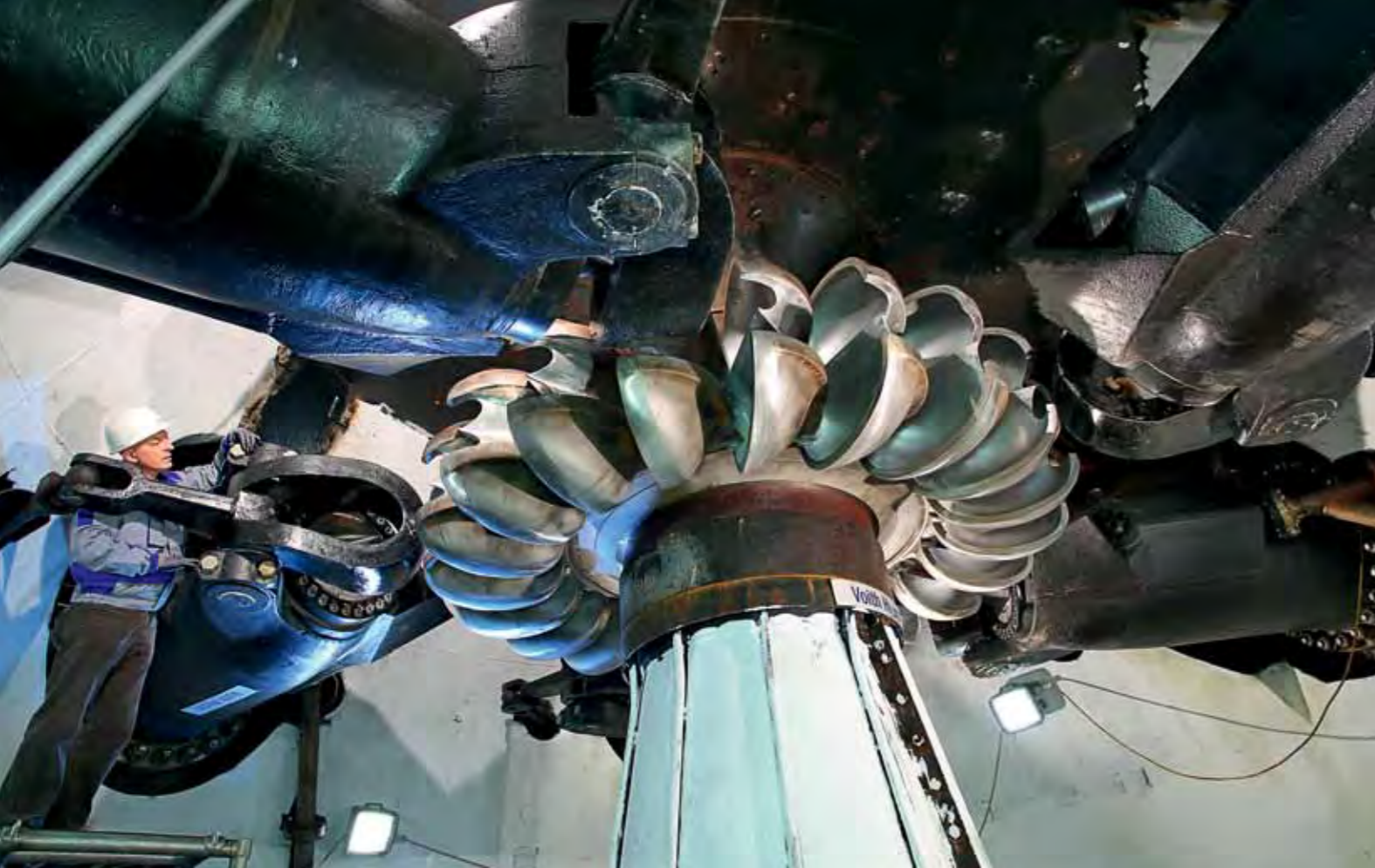
Pelton runner with modified Tosi injector, fully assembled after revision and ready for commissioning.
