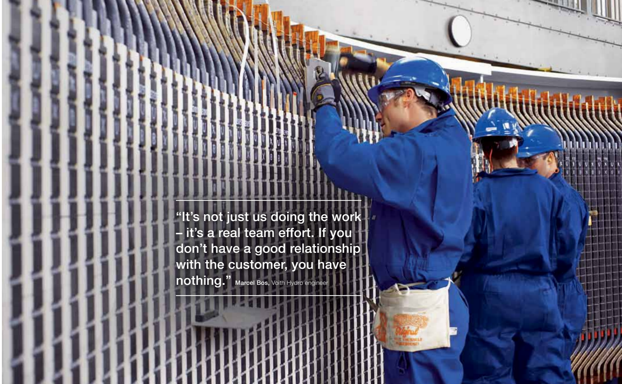
Modernization work on generators can help extend a plant's life span by decades.
