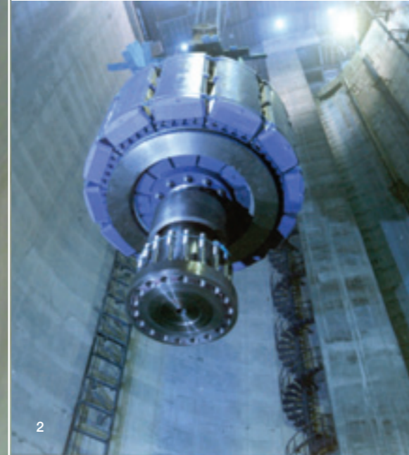
1-2 Stator and Rotor installation during repair of Generator at site
