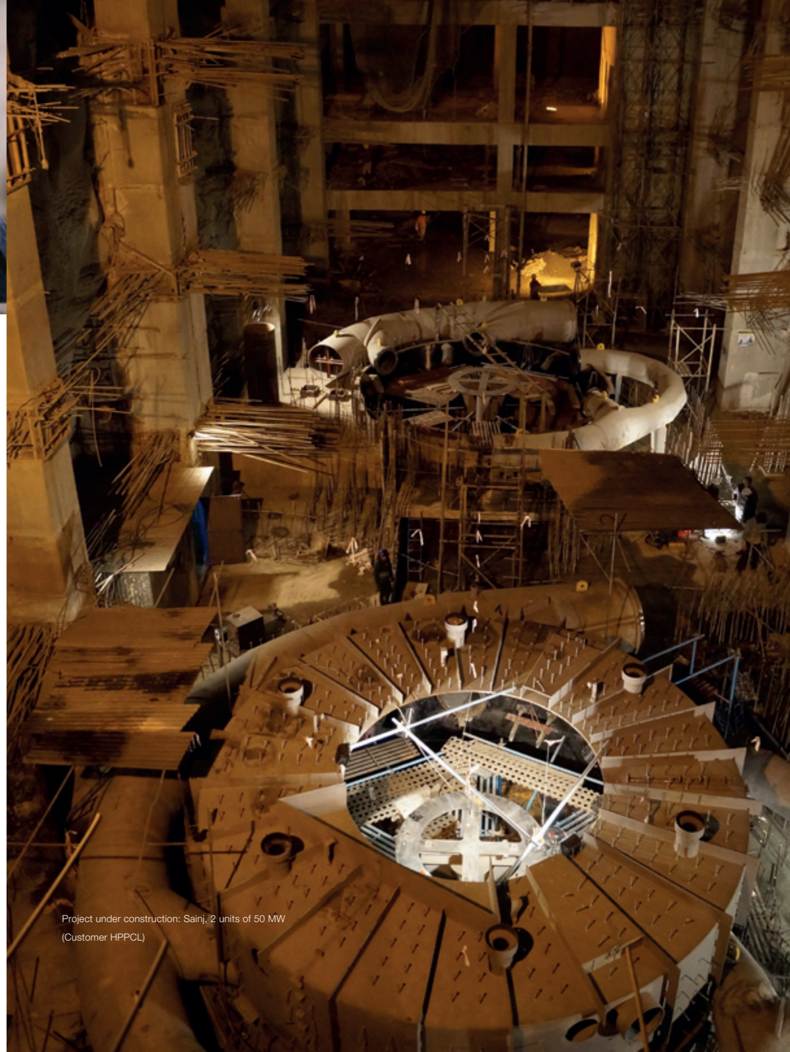
1 Stator assembly at Omkareshwar project, India 2 A proud worker at the Omkareshwar site
