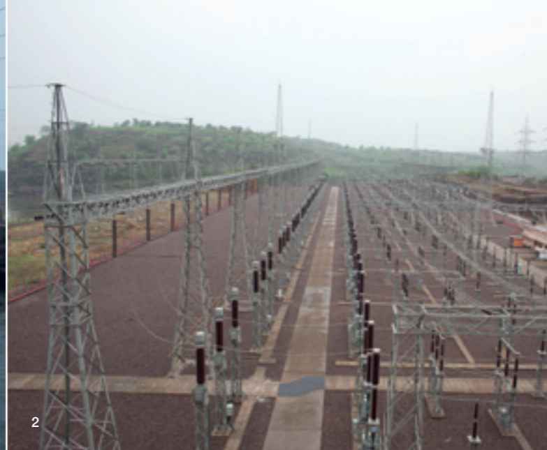
1 Omkareshwar Project 2 A massive 220 kV, 15 bay out door switch yard
