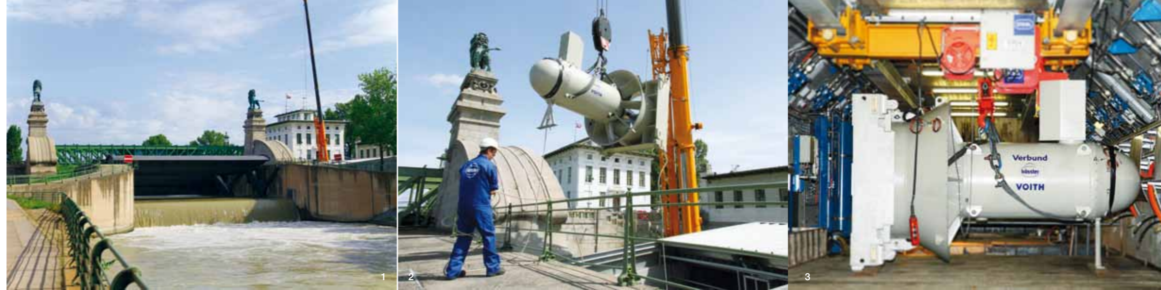
1 Historic Nussdorf site near Vienna, Austria 2 StreamDiver unit during installation 3 StreamDiver in service position
