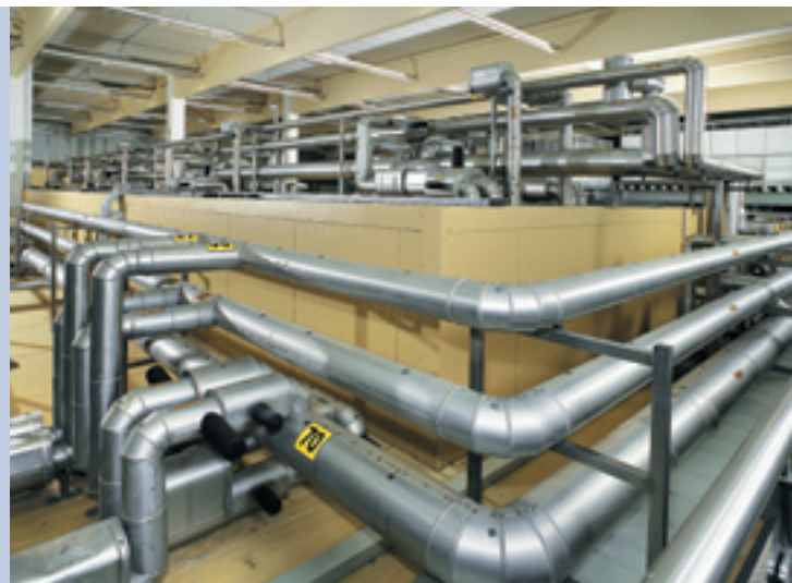
Cooling tunnel (exterior view)
