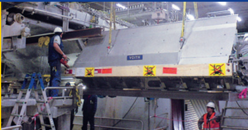
The installation of the back ply headbox was a real challenge
