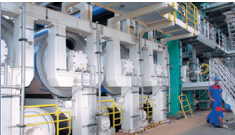
The dryer of the new board machine in Monte Alegre
