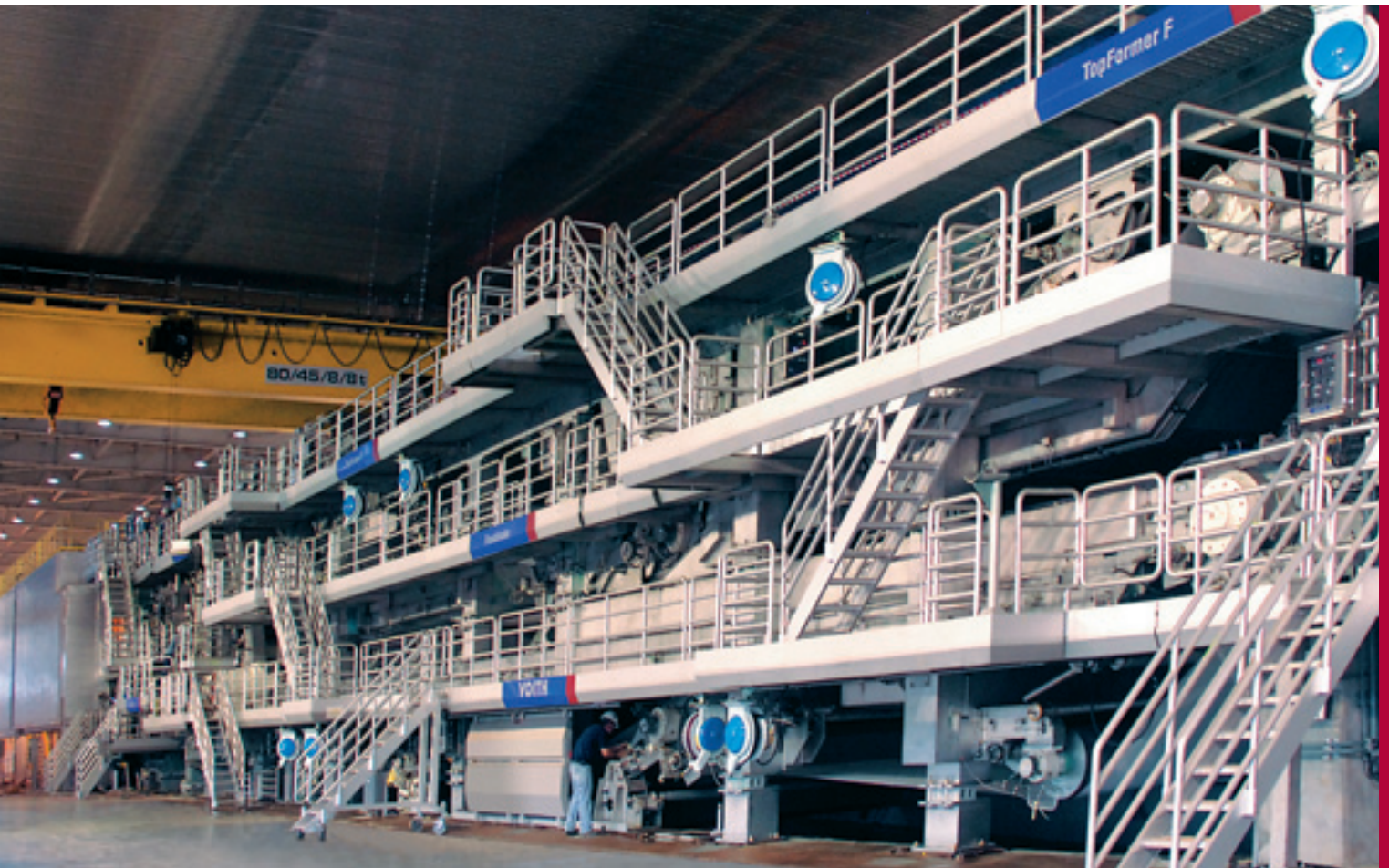
The new paper board machine from Voith on Monte Alegre is almost 240 meters long
