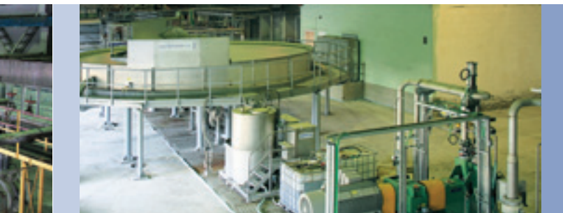
The same view after rebuild, with new refiners and additionally installed water treatment
