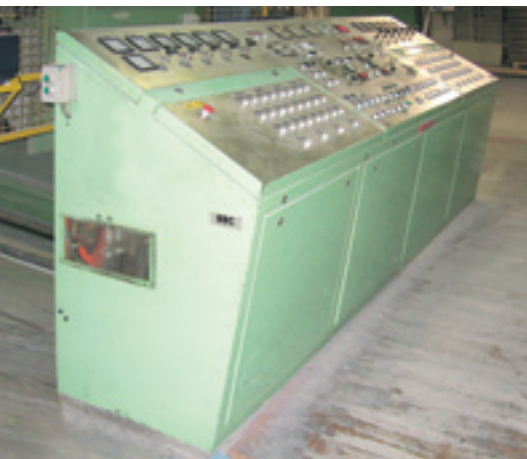
Control desk prior to rebuild
