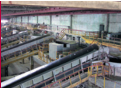
Charging zone before and after the rebuild
