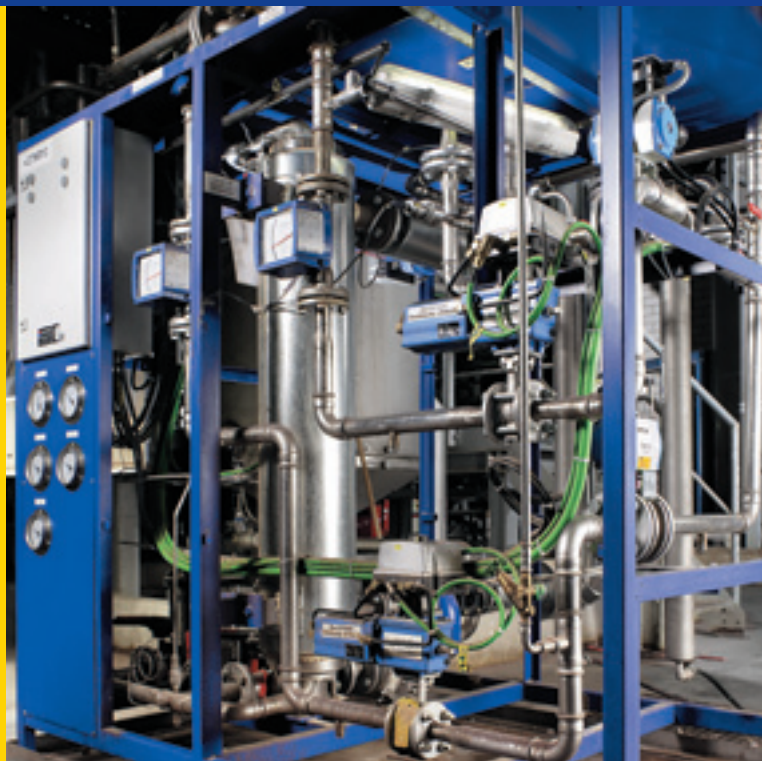
Water station for supply of ModulePro C
