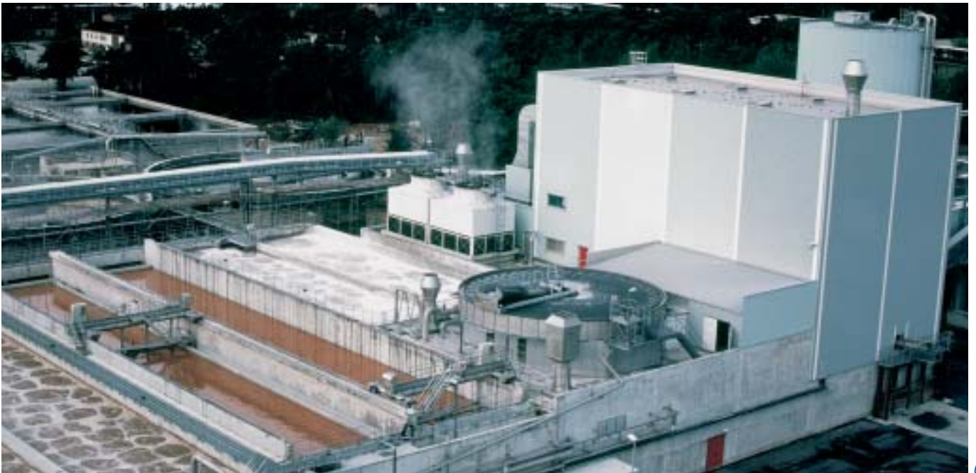
Fig. 7: Microflotation used for loop clarification and filtrate thickening in a deinking plant.
