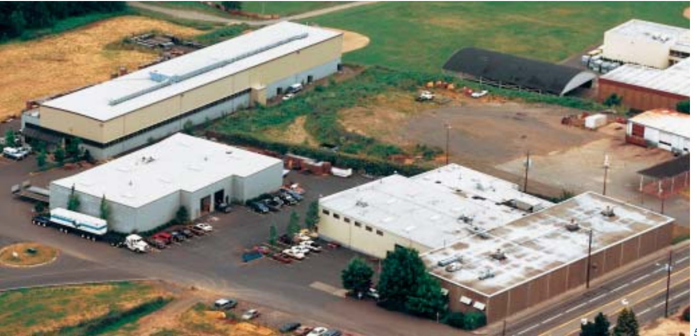
Fig. 6: VSWM – West Monroe, Louisiana.
