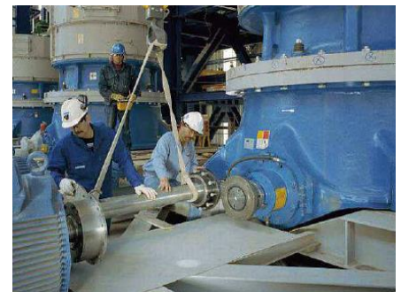
Installation of Voith SafeSet coupling with tooth connection coupling
