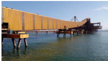
Loading & deloading terminal with conveyor belt
