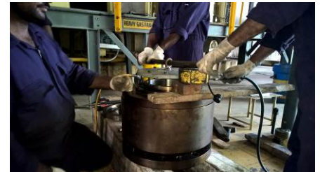
Removal of the spline sleeve of the SafeSet coupling by using 2 hydraulic jacks
