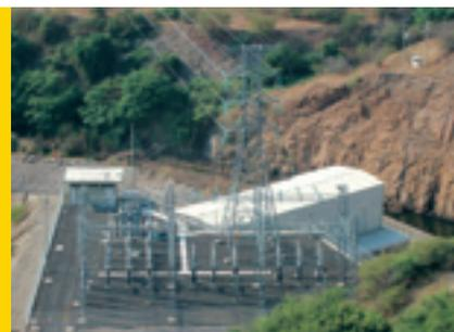
The Chilatán small hydro plant, owned by PEO – Provedora de Eletricidade de Occidente S.A. de C.V., recently went on line. The US\$12 million of this EPC contract see the supply two 7 MW Francis turbines, including the power station design and construction.
