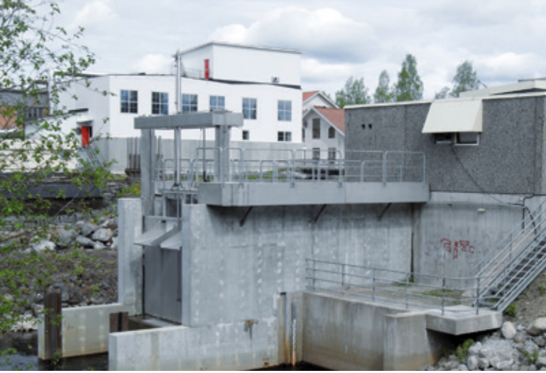
Bruksfors, Sweden: StreamDiver installation in existing power house
